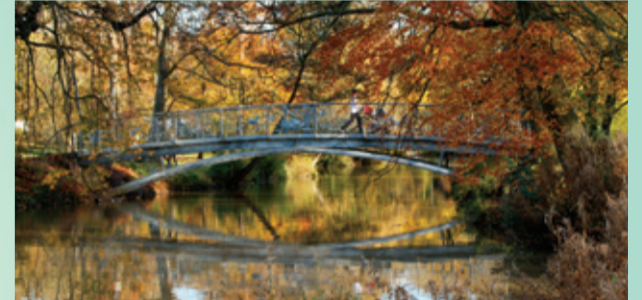
The Community Bridge opened in 2012
